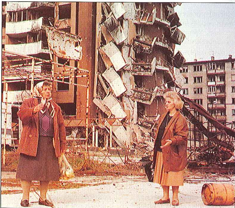
These two women stand in front of a building that has been heavily damaged in the war. The building is in Sarajevo, Bosnia.
